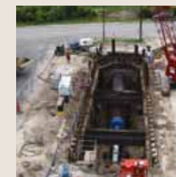
Horizontal pile driving
